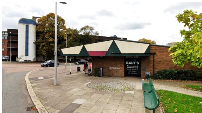
Figure 2. Flank elevation facing toward Little Park Street
