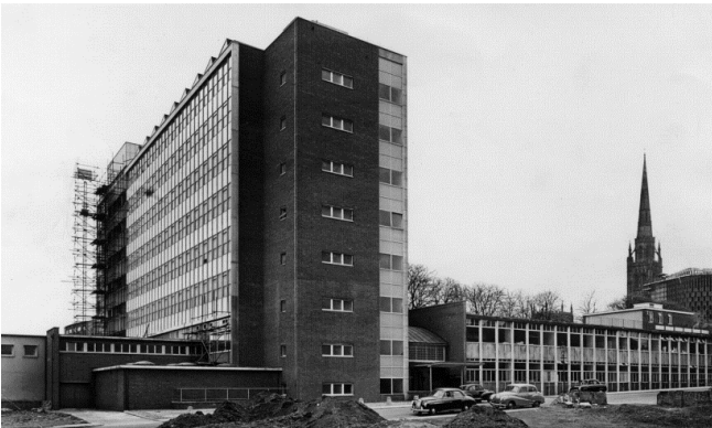
Figure 3. Final construction phase of the former Lanchester College of Technology in the 1960's known today as The Charles Ward building.
